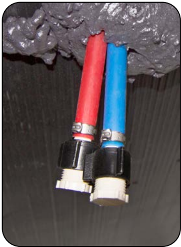
Low-Point Drain Valves located under the RV
