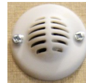
Typical temperature sensor (wall-mounted).
