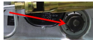
Typical anode rod, installed
