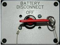
Typical battery disconnect switch
