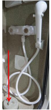
Typical outside shower. Remove the drain plug at the water hose access (indicated by the arrow) to allow excess liquids to drain out of the compartment area. This drain plug is NOT designed to sit flush with the compartment floor when inserted in the travel (and storage) position.
