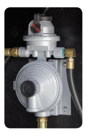
LP Regulator: The red color on the top dial indicates the LP bottles are empty. If the LP bottles were full, the dial would show green. When there are double cylinders on your RV, use only one at a time. Otherwise, the propane supply will be drawn equally from both cylinders until the supply has been exhausted. Using one cylinder until it is empty, before using the second, allows you to fill the empty cylinder at your convenience without running out of propane.
