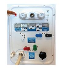
14. Turn **BLUE**, **GREEN** and **WHITE** handles so they are at a 45 degree angle for 10 seconds as shown.
