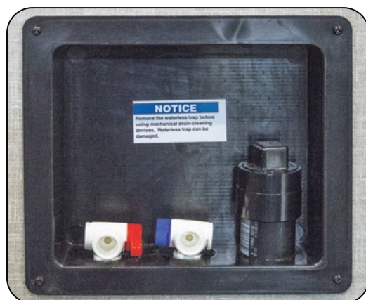
Hot & Cold Water Washer Hookups
