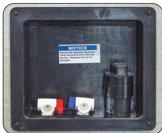
Hot & Cold Water Washer Hookups
