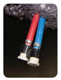
Low-Point Drains located under the RV
