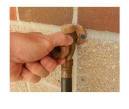
7. Disconnect garden hose from **"TANK FLUSH"** inlet.
