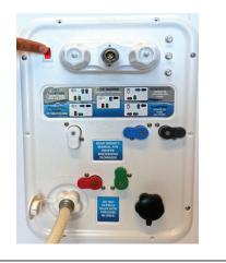
14. Turn **BLUE**, **GREEN** and **WHITE** handles so they are at a 45 degree angle for 10 seconds as shown.
