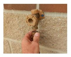
7. Disconnect garden hose from **"TANK FLUSH"** inlet.
