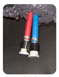
Low-Point Drains located under the RV
