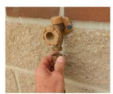
10. Disconnect garden hose at source before disconnecting from Nautilus panel.
