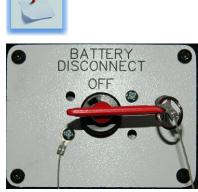
Typical battery disconnect switch
