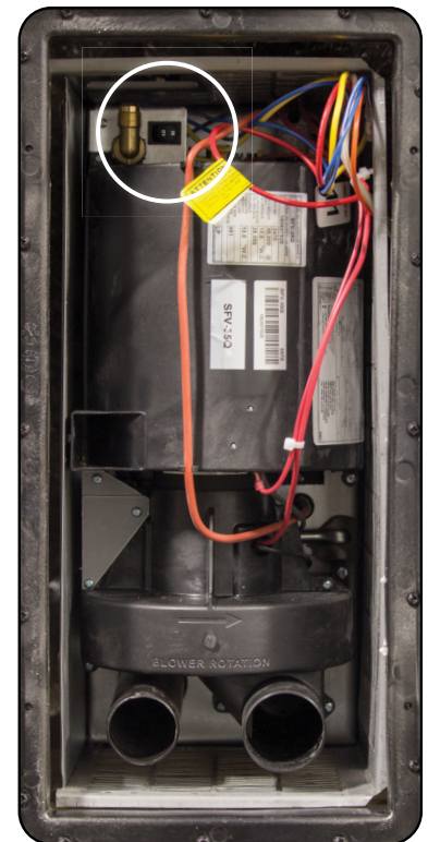
To Access the ON/OFF Switch, Remove the Outside Furnace Panel
