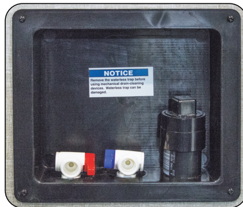
Hot & Cold Water Washer Hookups
