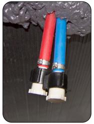
Low-Point Drain Valves located under the RV
