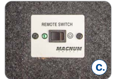
Inverter Remote Switch
