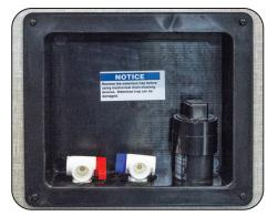
Hot & Cold Water Washer Hookups are typically located in the front bedroom or in the rear garage area.
