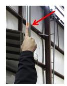
5. Finally, adjust the awning height, and slide the orange colored lock to secure each vertical awning leg in place as shown above.
