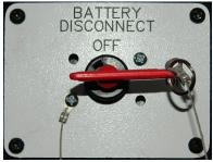
Typical battery disconnect switch
