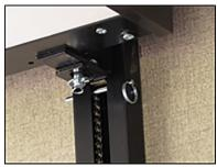
Photo shows typical Happijac© locking pins, with the top bed locked in the highest position
