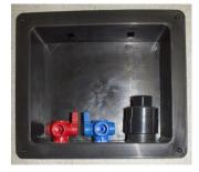
Washer hot and cold water hookups and drain, typically either located in the door-side front bedroom closet or in the rear garage area.
