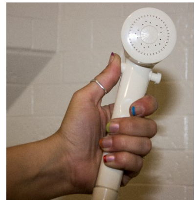
Typically, most RV bathroom shower heads have a shut off valve (as shown in the photo above for this particular model).
