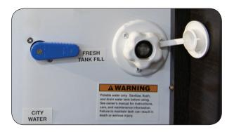
For normal city water use (for example, at a campground), turn the city water control handle as shown below:
