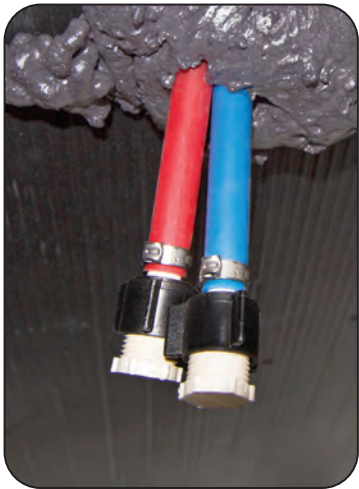
Low-Point Drain Valves located under the RV
